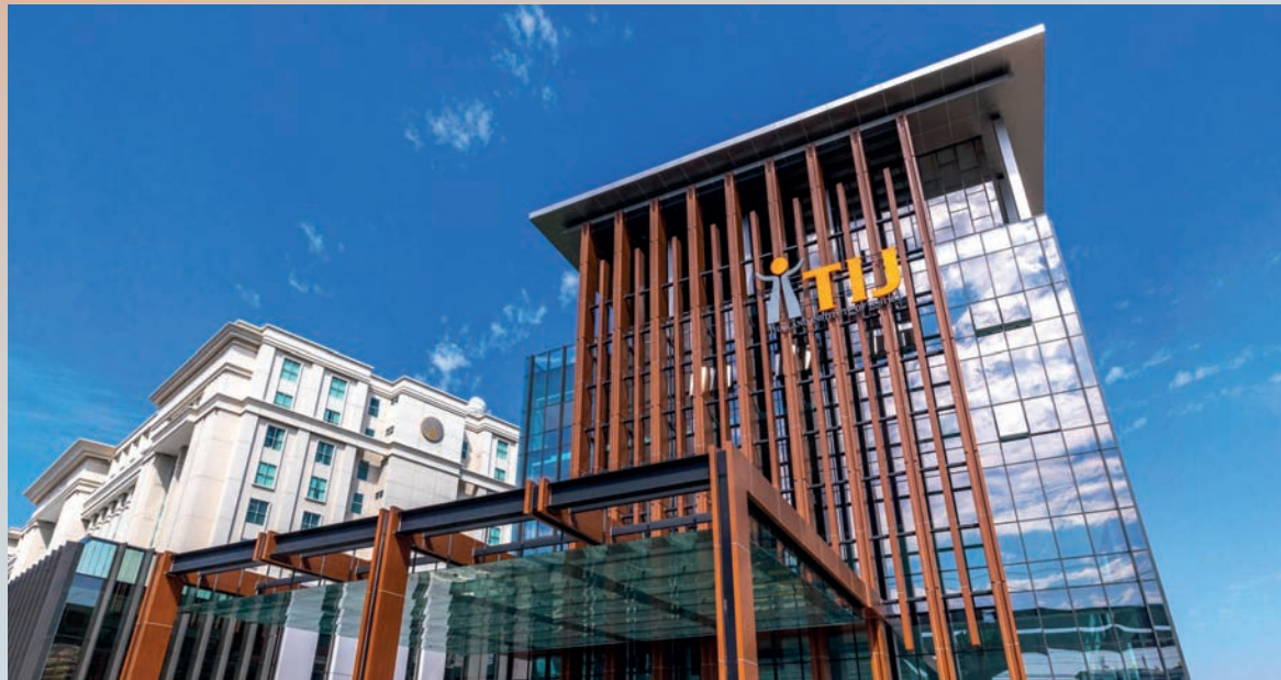
The new TIJ building next to the Ministry of Justice is located on Chaengwattana Road, Bangkok.
